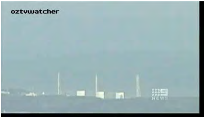
March 14, 11:00 No.3 reactor building hydrogen-exploded. (From Fukushima central television)
