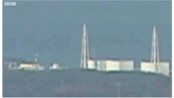
March 12 2011, 15:00 No.1 reactor building hydrogen-exploded. (From Fukushima central television)
