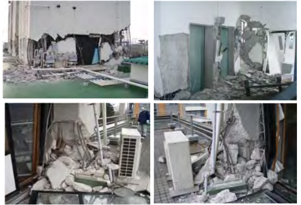
3 buildings of departments of electric engineering, architecture and civil engineering, and materials science and engineering were broken and now renewed.
